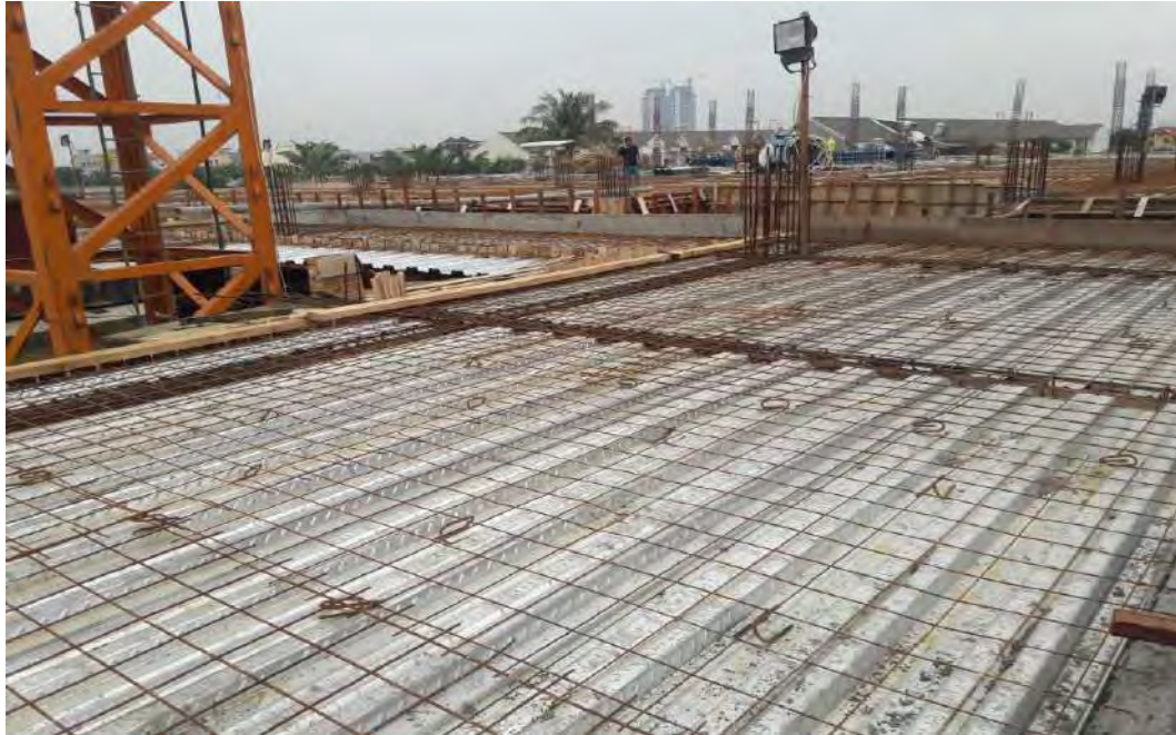
Gambar Bekisting Plat Lantai
