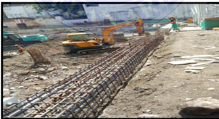
Gambar 4.5 Pembesian Capping Beam
