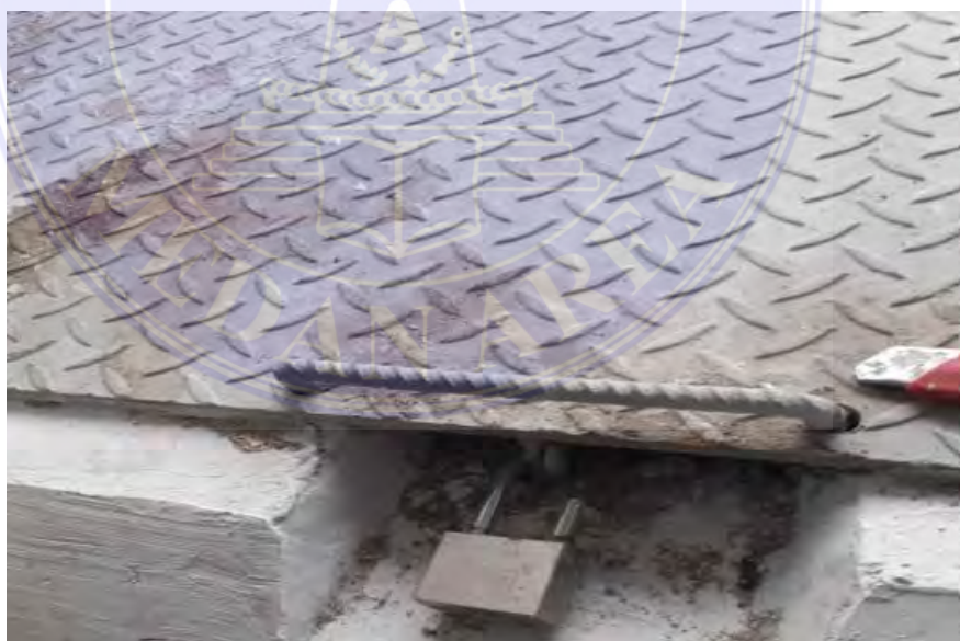
Gambar 6. Manhole Clean Water Tank (Amanda. Mutia. 2020)
