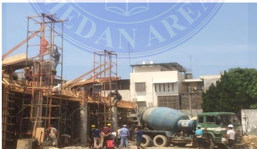
Gambar 3.9 Lift Beton
