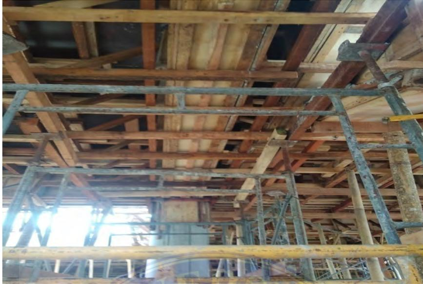
Gambar 3.23. Bekisting balok
