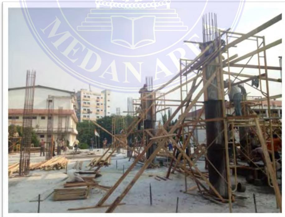
Gambar 8: Bekisting Kolom
