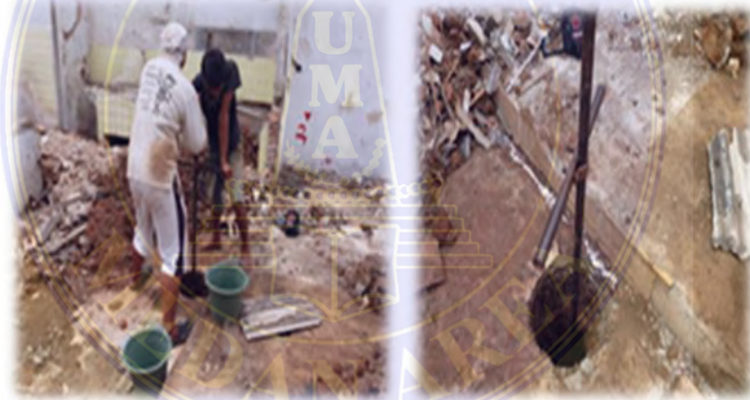
Gambar 2.5 Bore pile manual
