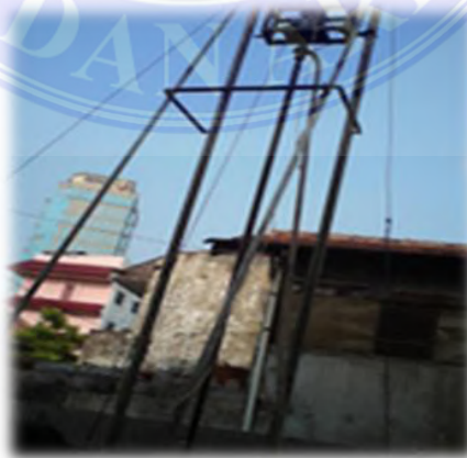
Gambar 2.4 Bore pile gawangan
