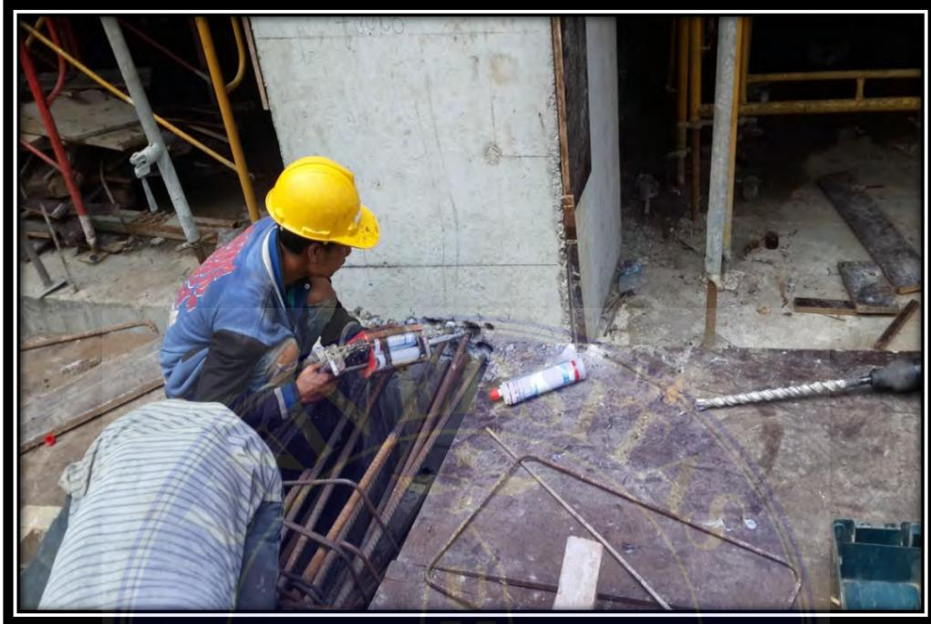
*Gambar 5. Chemical Anchor balok*
