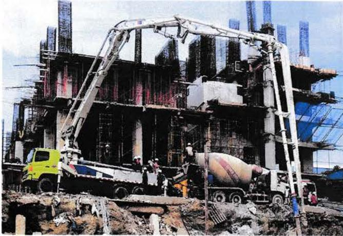
Gambar Concret Pump
