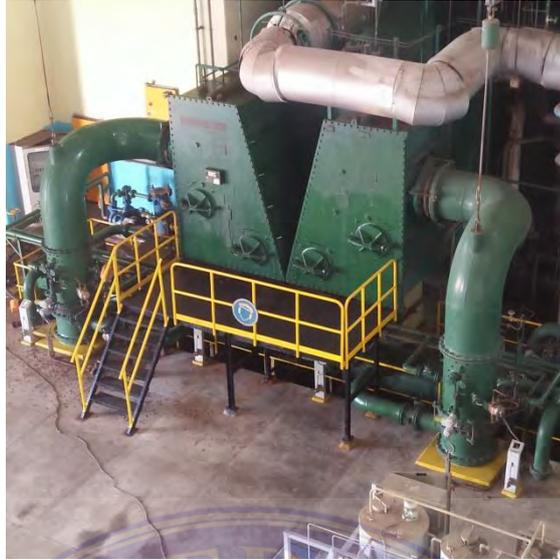
Gambar 3.6 *Condensor Tipe CV30+44-2-99-25250*
