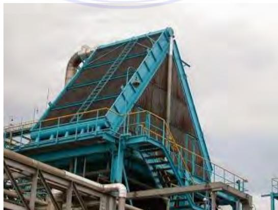
Gambar 2.12 *Air Cooled Condenser*
