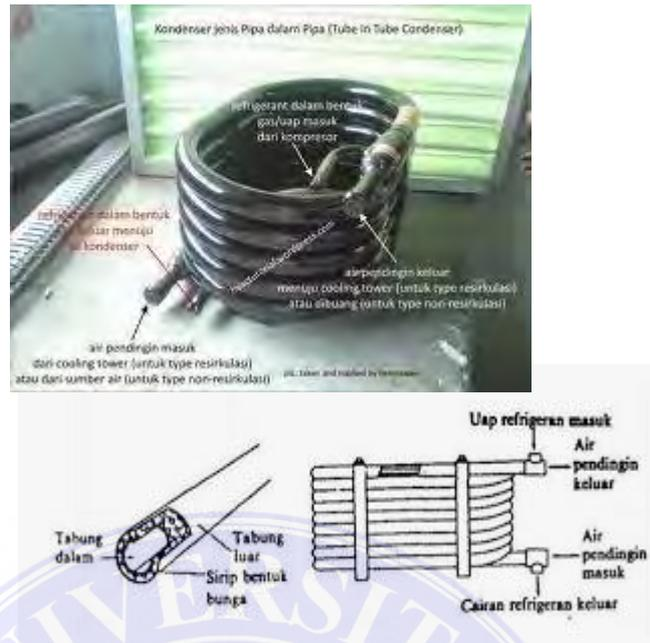
Gambar 2. 15 *Tube and Tubes Condenser*
