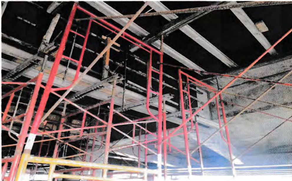
Gambar 5.4 Scaffolding Lantai Sumber : Data lapangan ,2016
