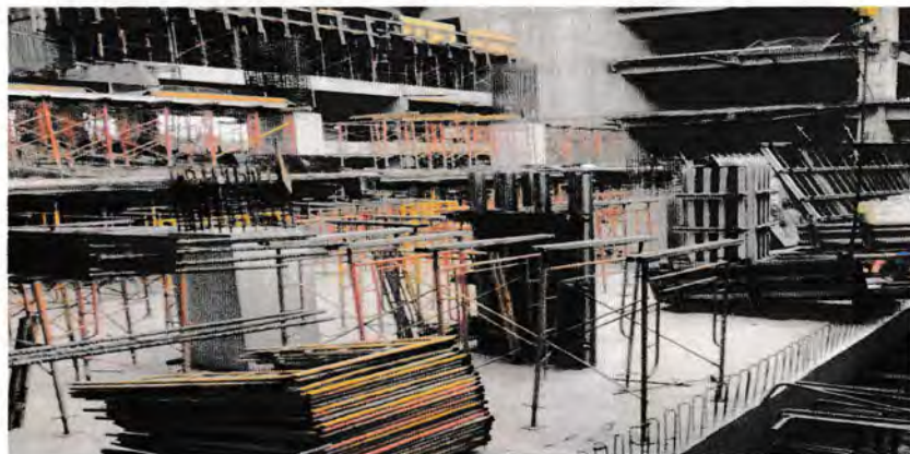
Gambar 4.11 Scaffolding Sumber : Data lapangan ,2016
