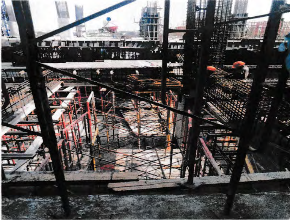
Gambar 5.3 Scaffolding Lantai Sumber : Data lapangan ,2016
