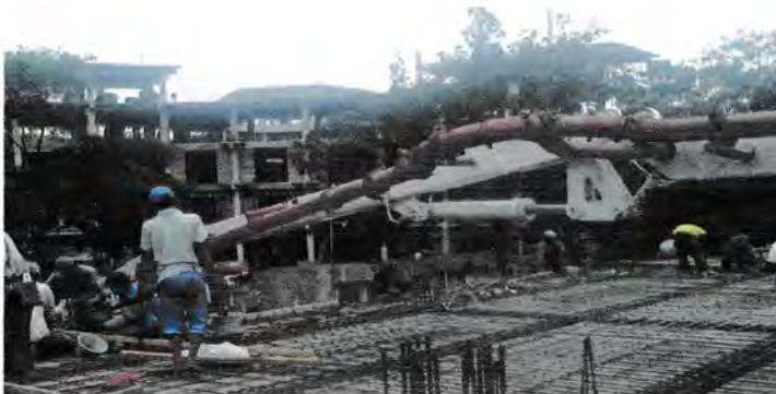
**Gambar Pump Concrete**
