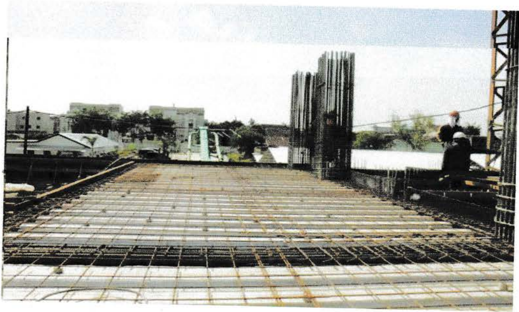
Gambar 9 : Wiremesh Lantai 2
