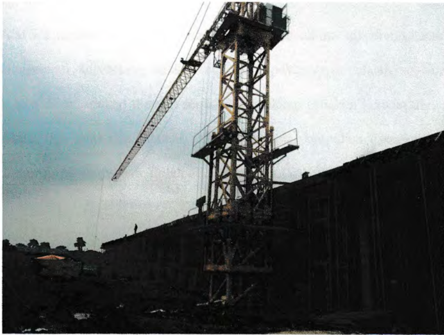
Gambar 2.2g: Tower crane (proyek Mall of Metrolink Trade Center)
