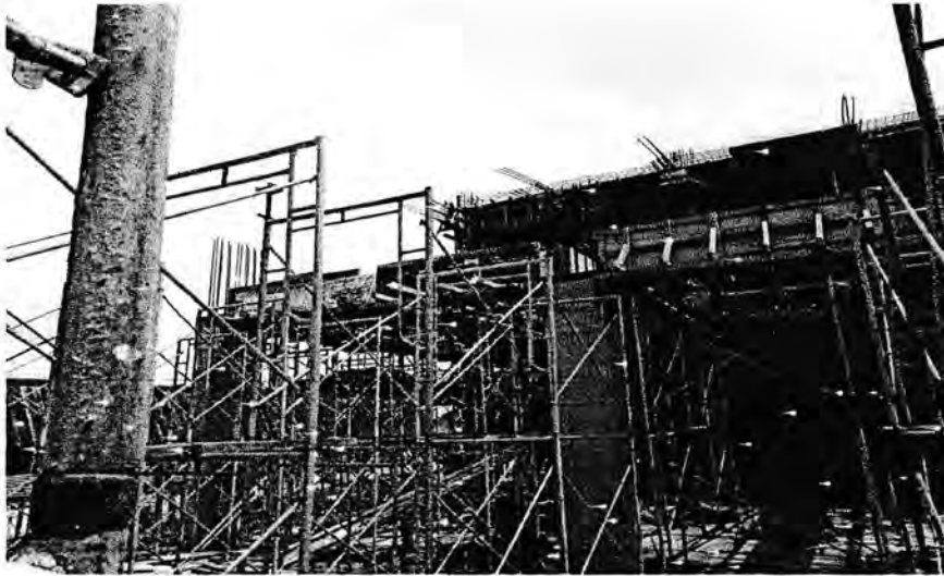
Gambar 3.15 Bekisting balok
