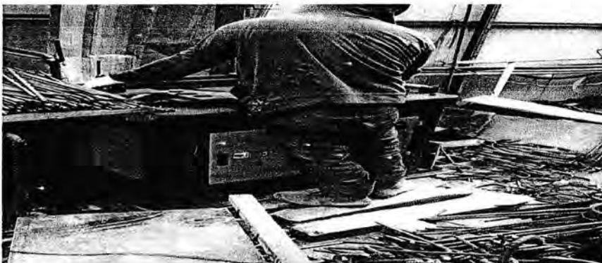
Gambar 3.5 Bar Bending
