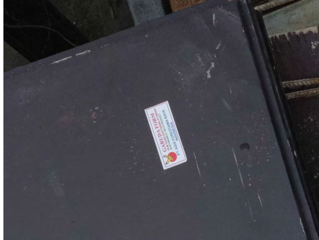
Gambar 2.23 (c) 2 film faced plywood 12 mm.
