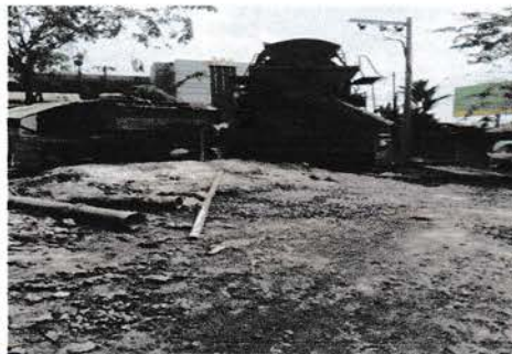
Gambar 3.3 : Beton ready mix
