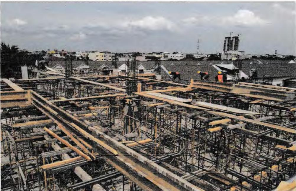
**Gambar 5.18 Bekisting Balok**
