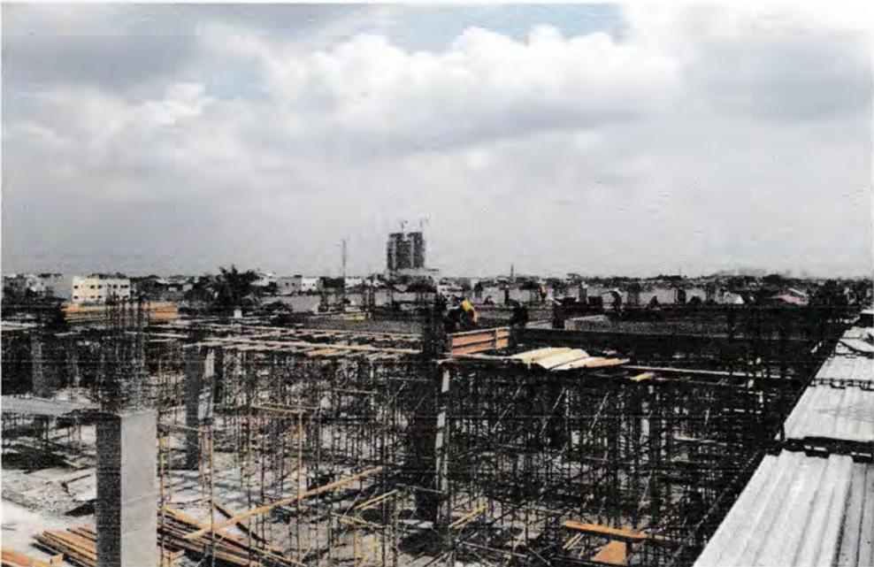
**Gambar 5.16 Bekisting Balok**
