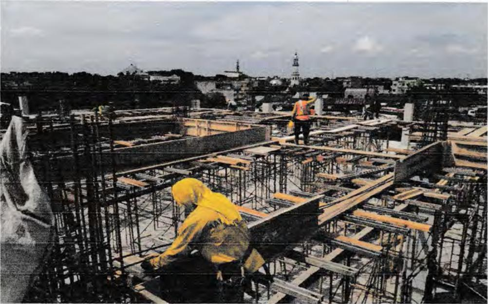
**Gambar 5.17 Bekisting Balok**
