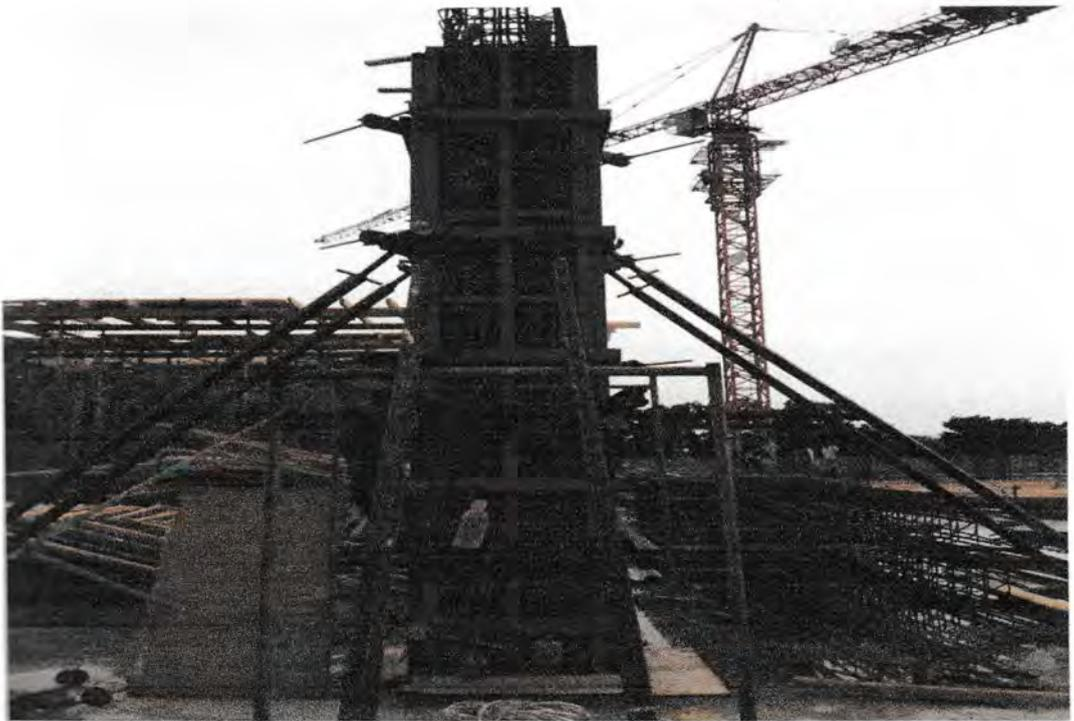
**Gambar 4.9 bekisting kolom**
