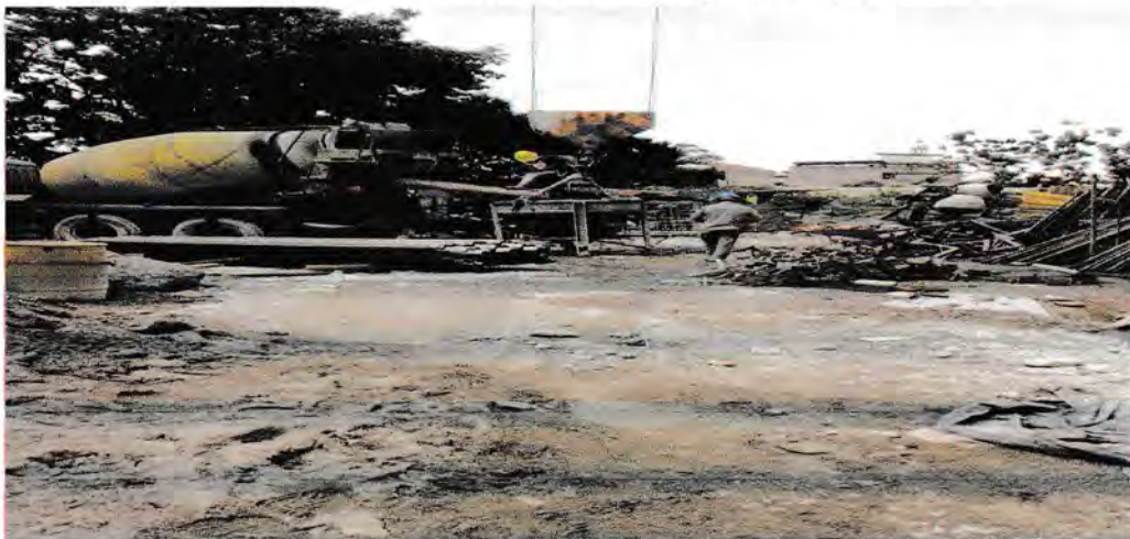
Gambar 4.1 Beton Ready Mix
