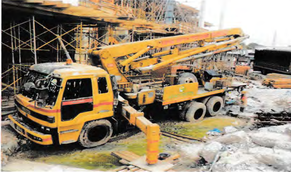
Gmabar 4.2 Pump Concrete
