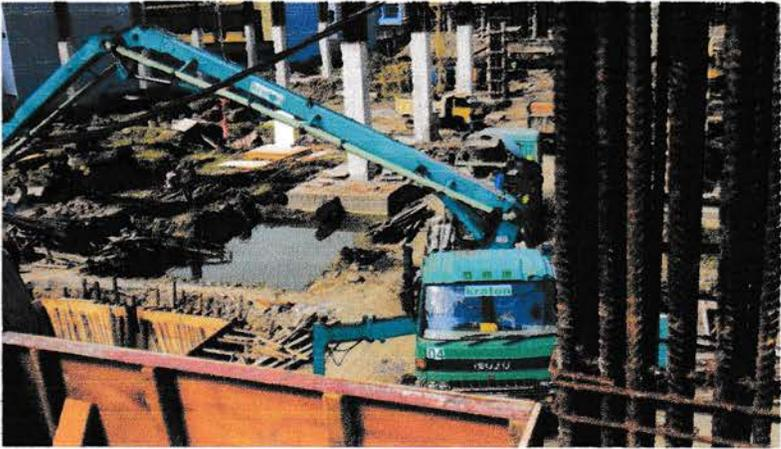
Gambar 4.2. Pump Concrete
