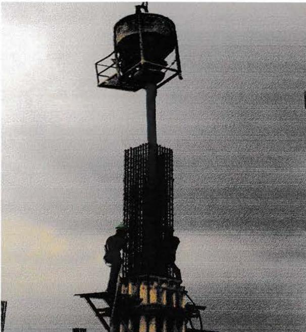
Gambar 4.8. Bucket Cor (Concrete bucket)
