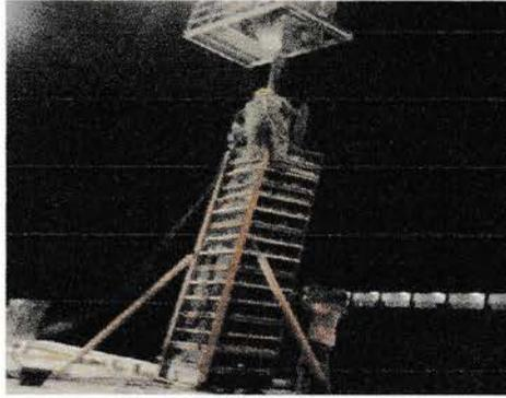
**Gambar 3.1. Bekisting kolom (bekisting dinding peri)** (Sumber : Data Lapangan 2016)
