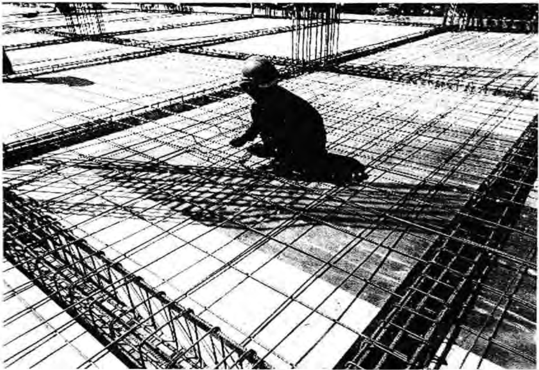
Gambar 3.3. Bekisting plat lantai
