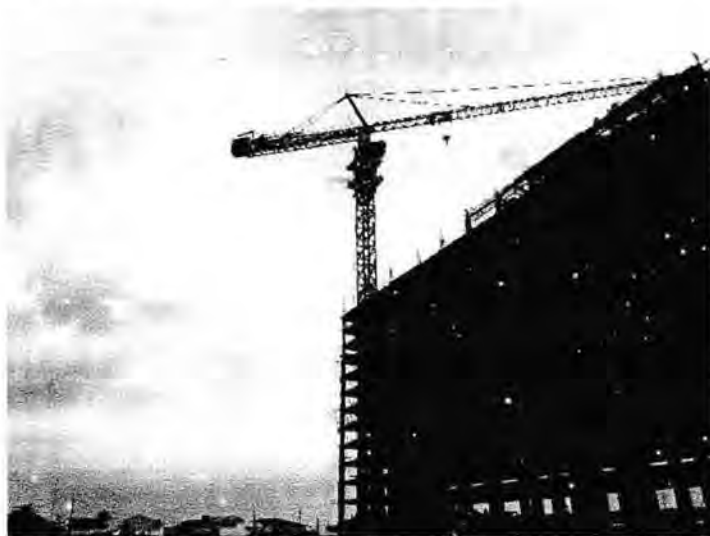
Gambar 4.8 Tower Crane Sumber: Data Lapangan 2016
