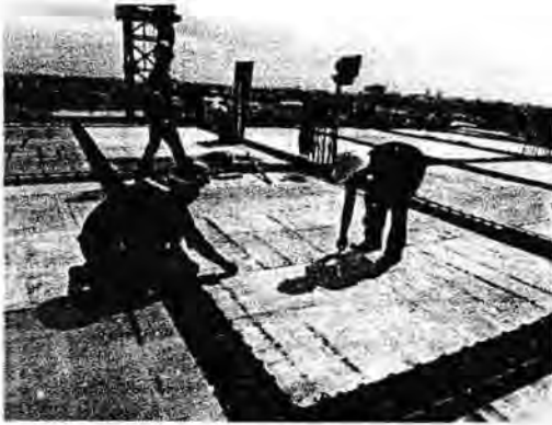
(c) Proses marking bekisting lantai
