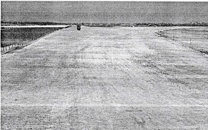
Gambar 3.2 : Lapisan CTB (Cement Treated Base)
