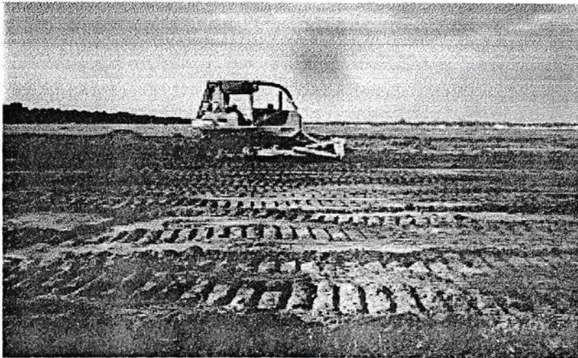
Clearing/ Stripping Taxiway
