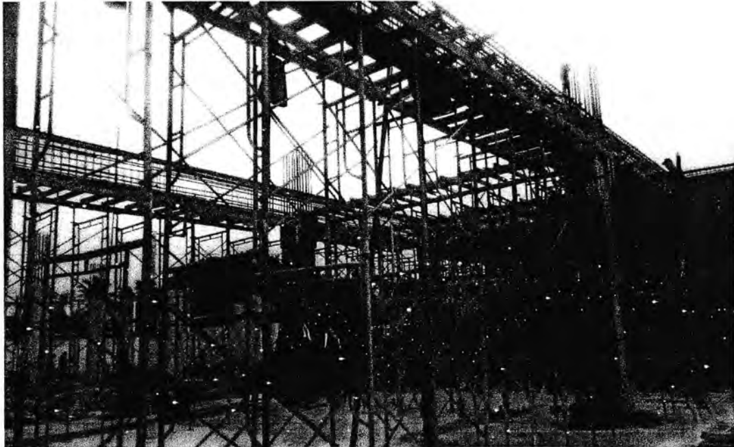
Gambar 3.18 Bekisting balok
