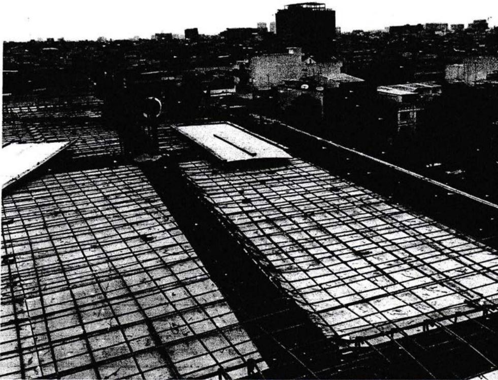
Gambar 3.20 Bekisting plat lantai
