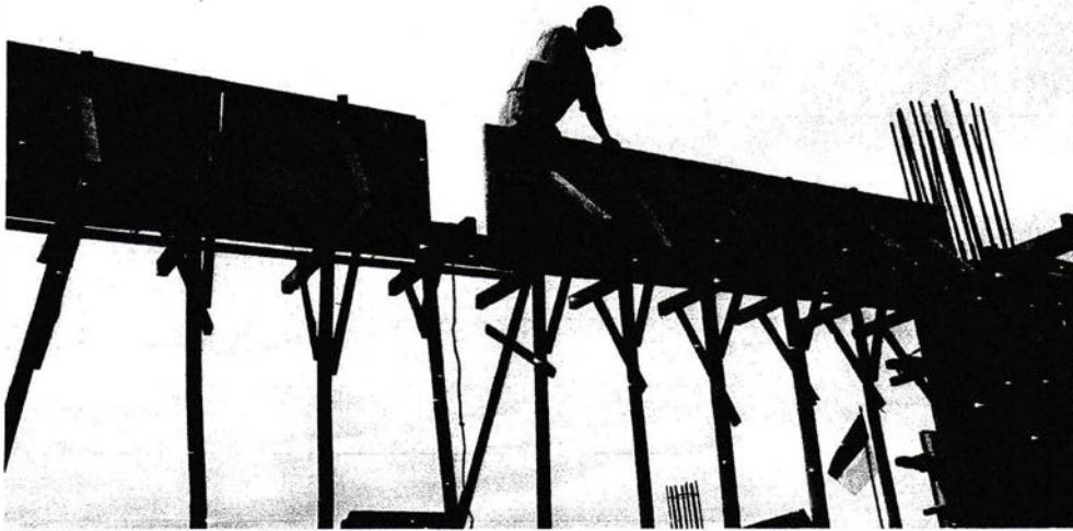
Gambar 3.19 Bekisting balok
