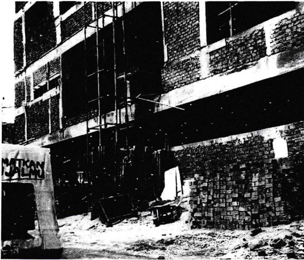
Gambar 3.5 Lift Beton
