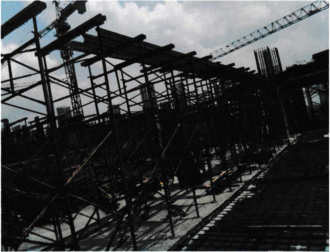
Gambar 5.9 Scaffolding Balok Sumber : Data lapangan ,2016
