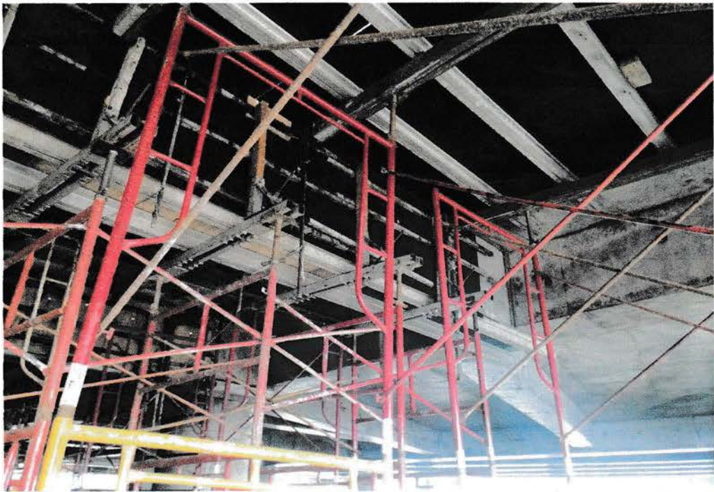
Gambar 5.4 Scaffolding Lantai Sumber : Data lapangan ,2016
