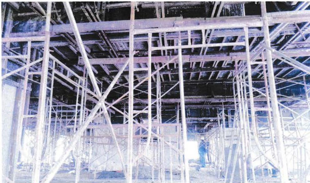
Gambar 3.12 Scaffolding Sumber : Data lapangan ,2017
