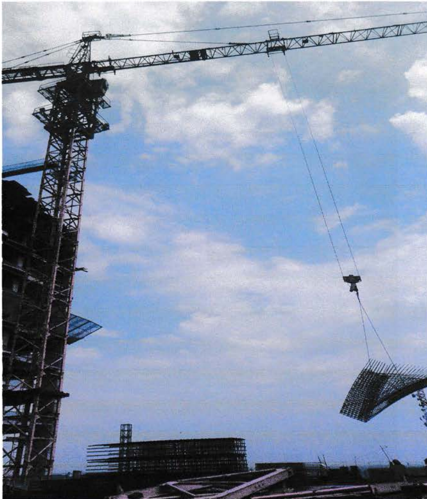
Gambar 3.9 Tower Crane Sumber : Data lapangan ,2017
