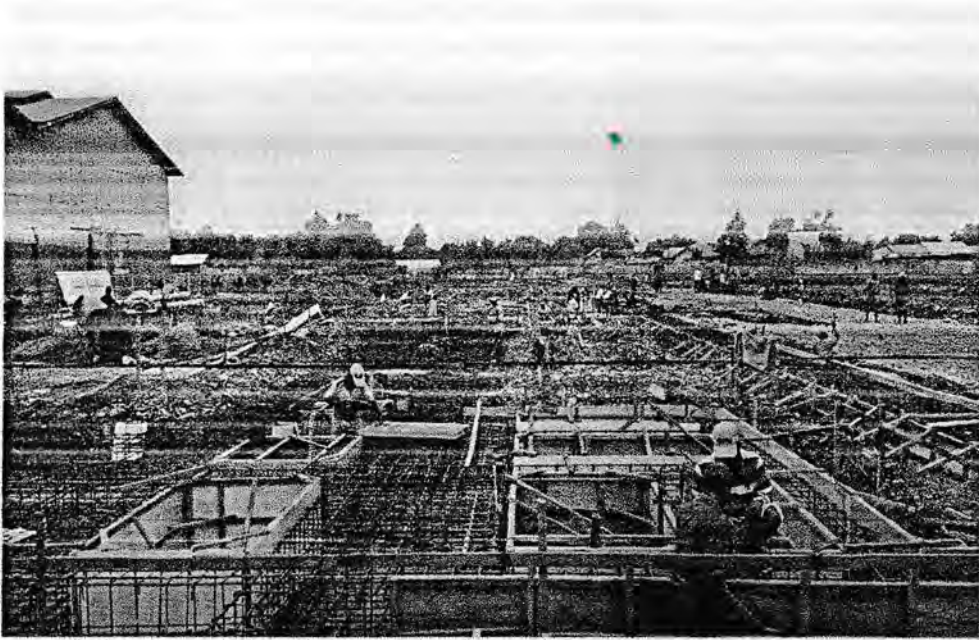
Foto Pemasangan Bow Plank Form Work Girder
