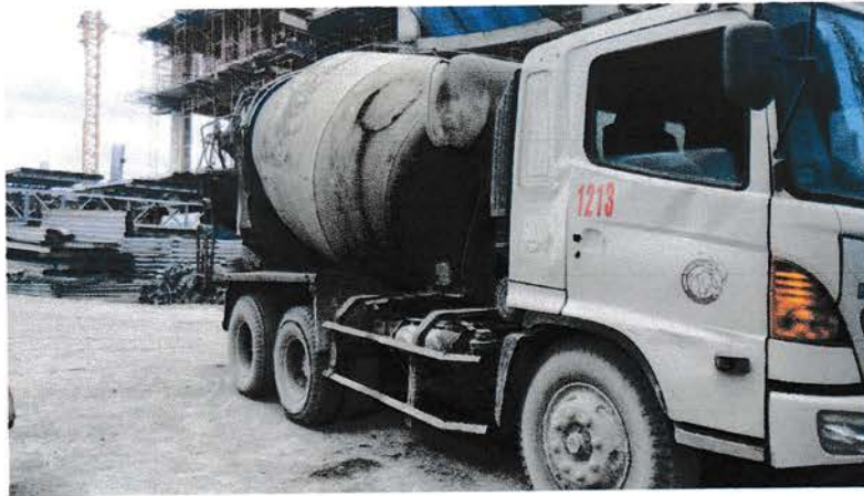
Gambar 3.2 Beton Ready Mix
