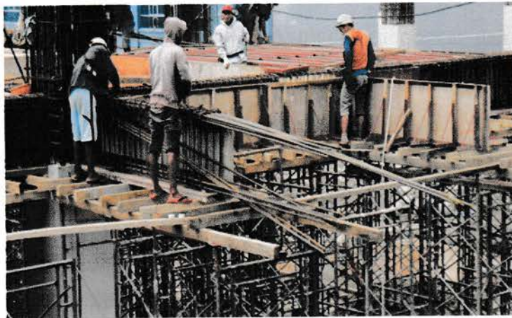
Gambar 3.16 Bekisting balok
