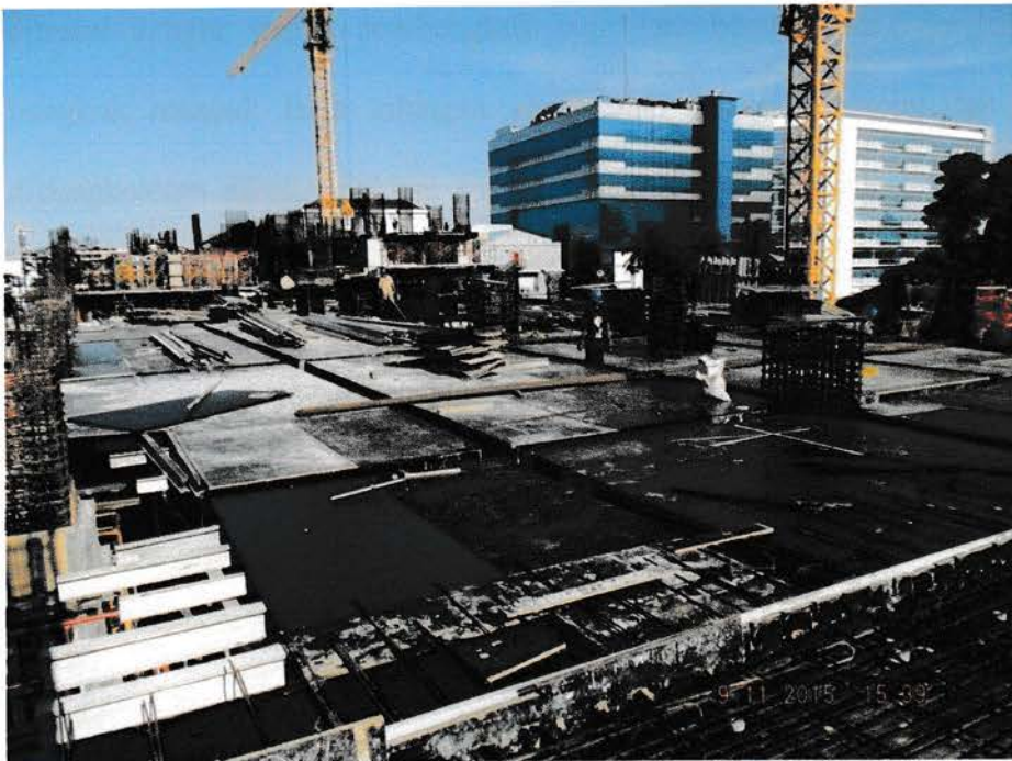
Gambar 3.17 Bekisting plat lantai
