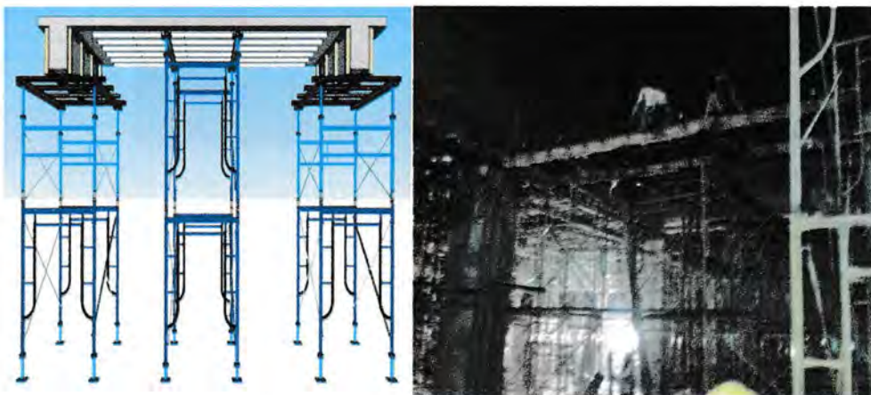
Gambar 3.2. Bekisting balok
