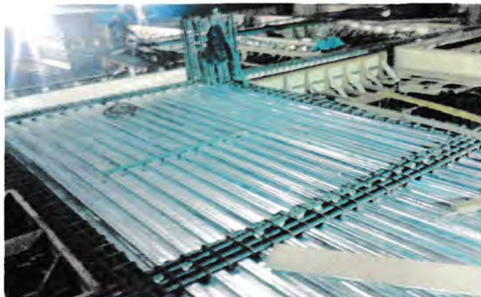
Gambar 3.3. Bekisting plat lantai
