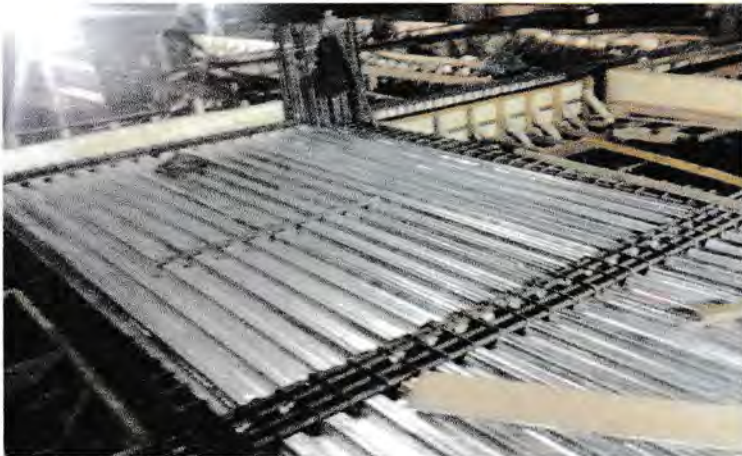
Gambar 3.3. Bekisting plat lantai
