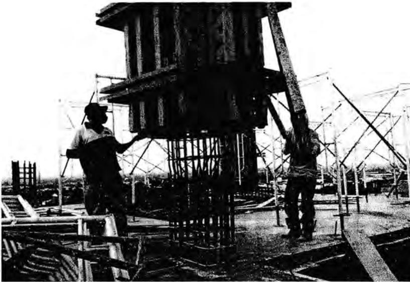
Gambar 3.19 Bekisting kolom
