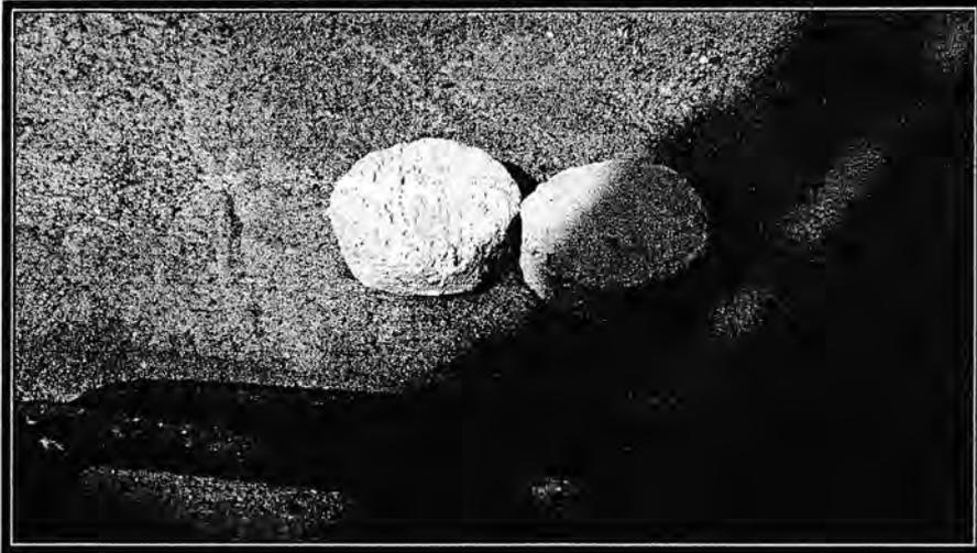
**Gambar 4.15 Beton decking**
