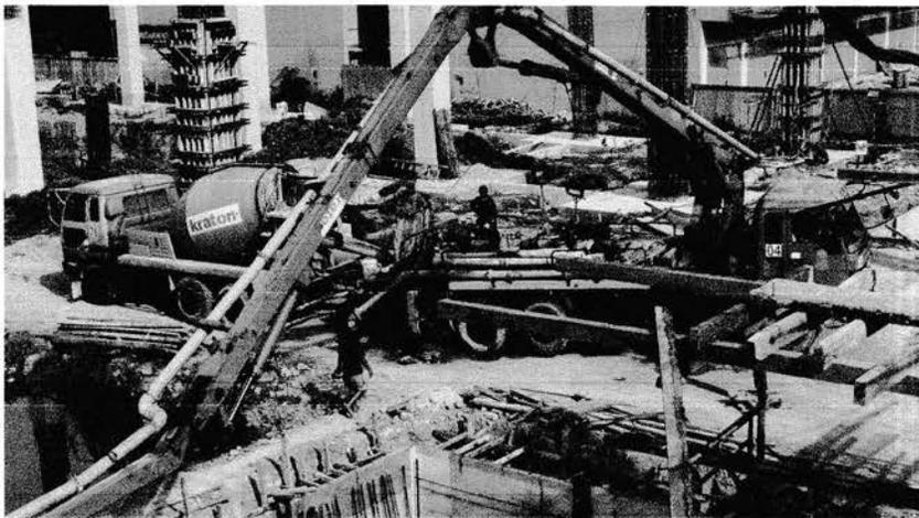
Gambar 4.16. Concret Pump
