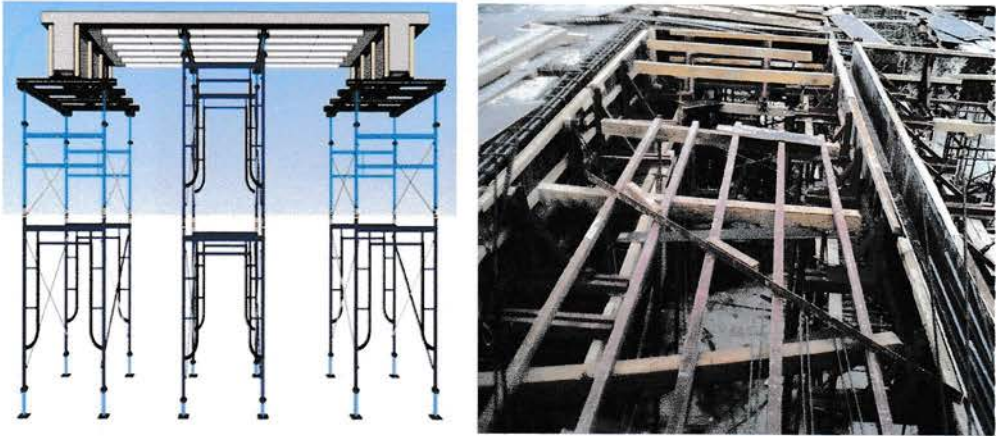
Gambar 3.2. Bekisting Balok
