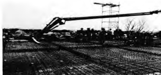
Gambar Pump Concret
