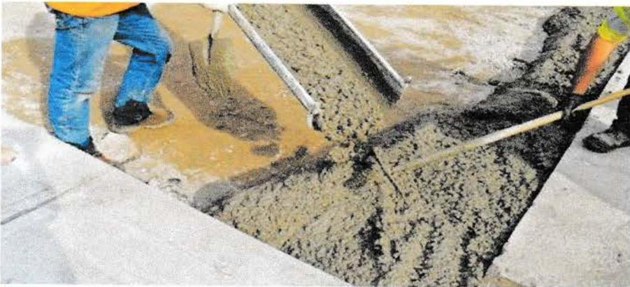
Gambar 2.1 Beton Ready Mix
