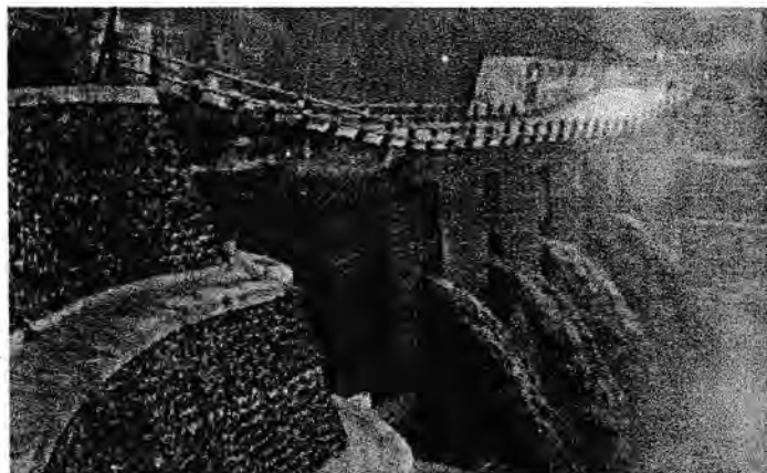
Gambar 2.2 Sabo Dam Gunung Merapi, Yogyakarta
