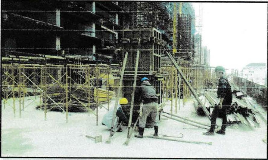
*Gambar 15. Menyetel Bekisting Kolom*
