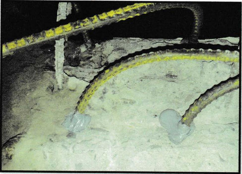
*Gambar 5. Chemical Anchor Pada Slab Lantai*
