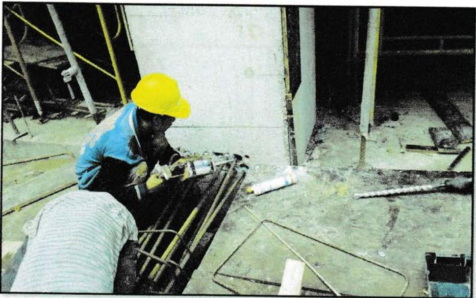
*Gambar 2. Chemical Anchor Balok*
