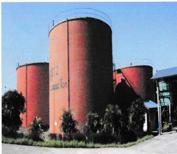
Gambar 39. Storage tank (ST)
