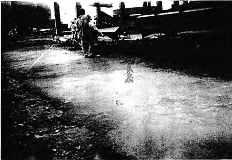
Gambar III.3. Pekerjaan lapisan pondasi (base course)
