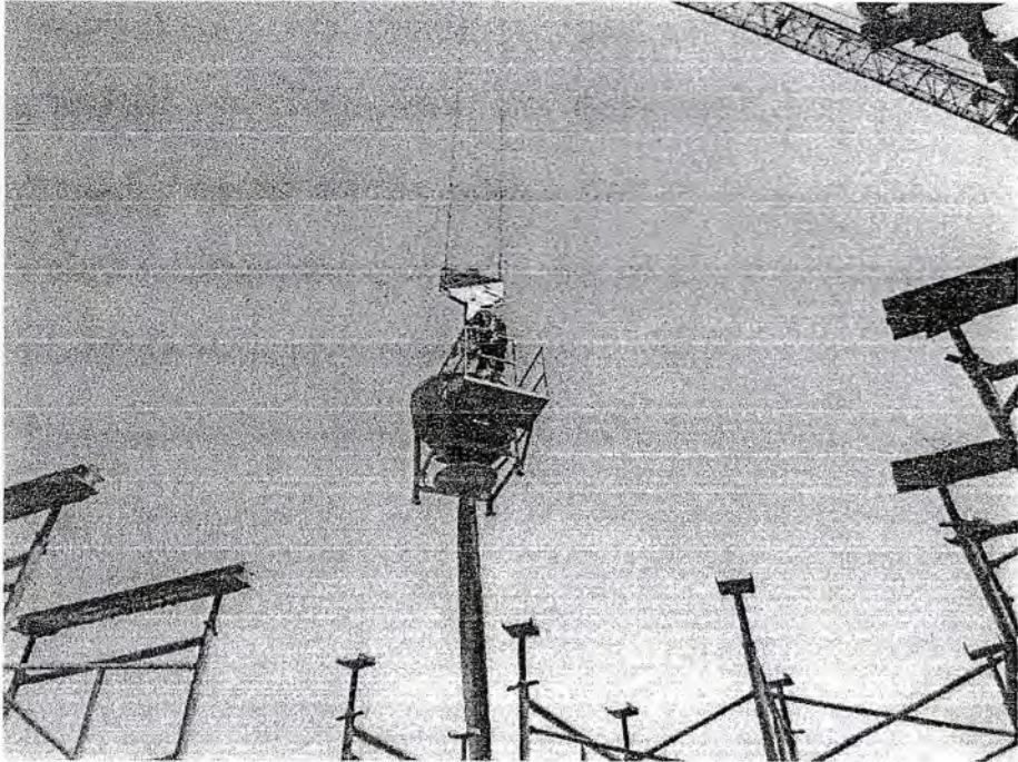
Gambar 4.3. Pengangkutan concrete bucket beserta operator
