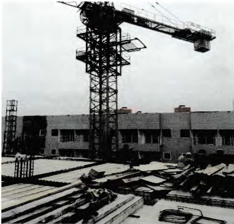
Gambar : Tower Crane
