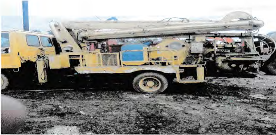
Gambar ; Pump Concrete
