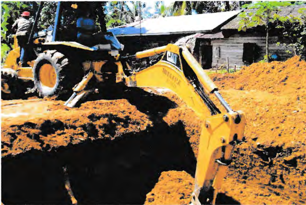
Gambar 2. Galian pondasi tower
