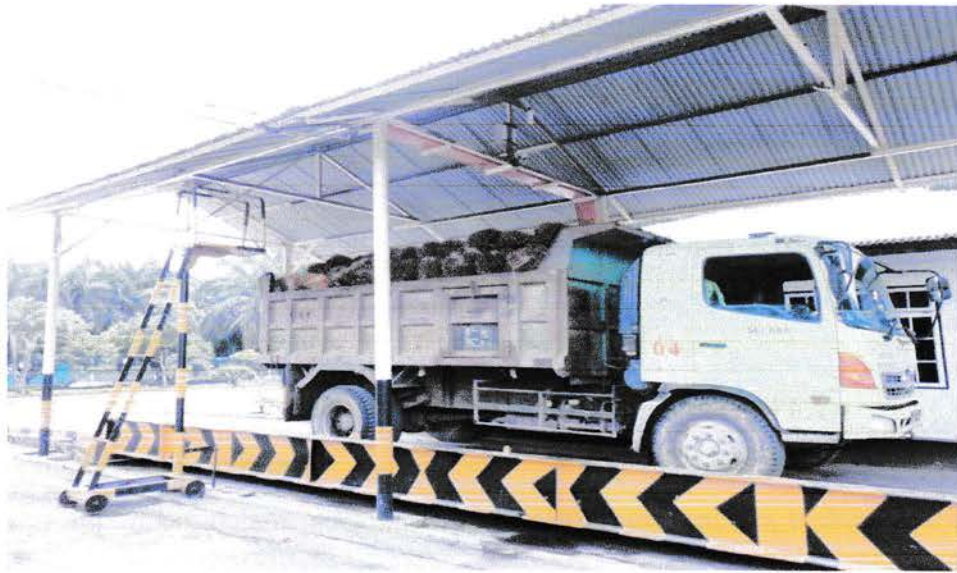
Gambar 11 : Pabrik Pengolahan Kelapa Sawit - Weighbridge/ Jembatan Timbang Loading Ramp
