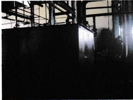
Gambar 14. oil transfer tank
