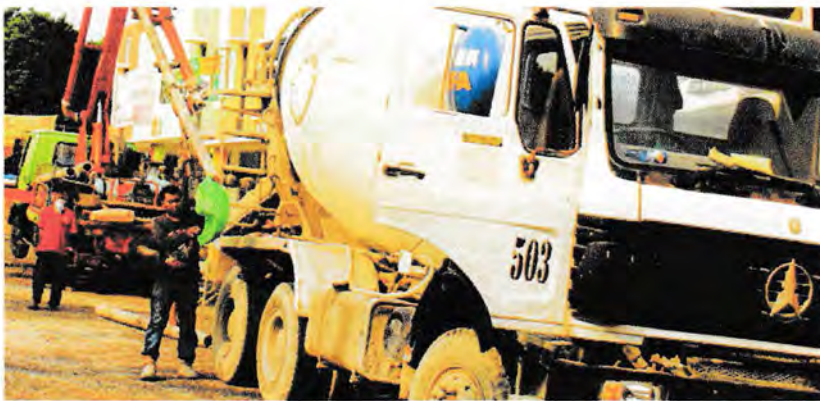
Gambar 3.1.2 Beton Redy Mix
