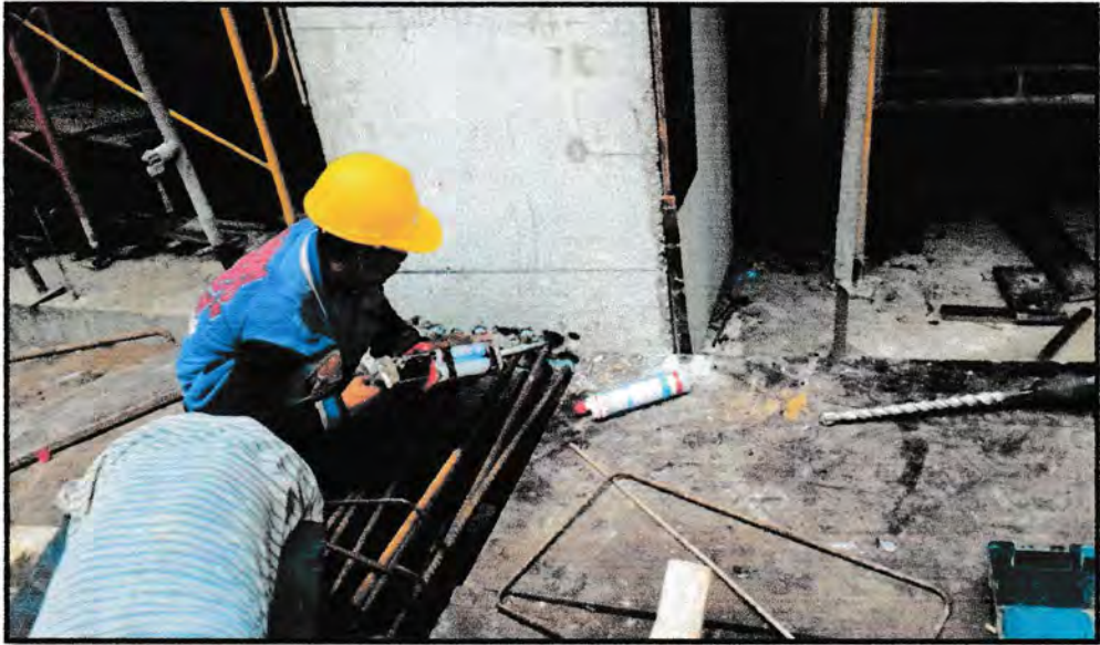
Gambar 5. Chemical anchor kolom
