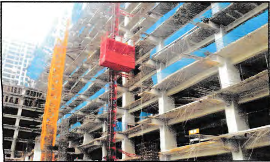
Gambar 3.2.7 Passenger Hoist (PH)
