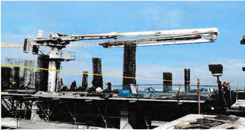
Gambar 3.2.3 Concrete pump
