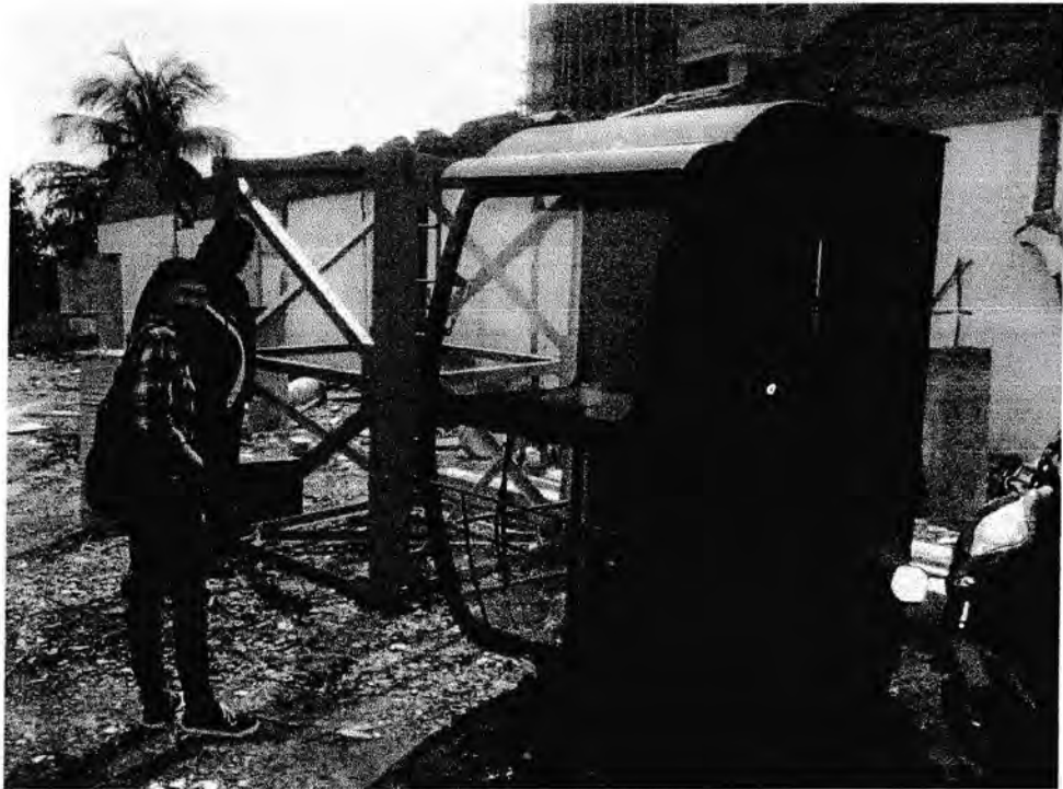
Gambar Tower craine sebelum dipasang
