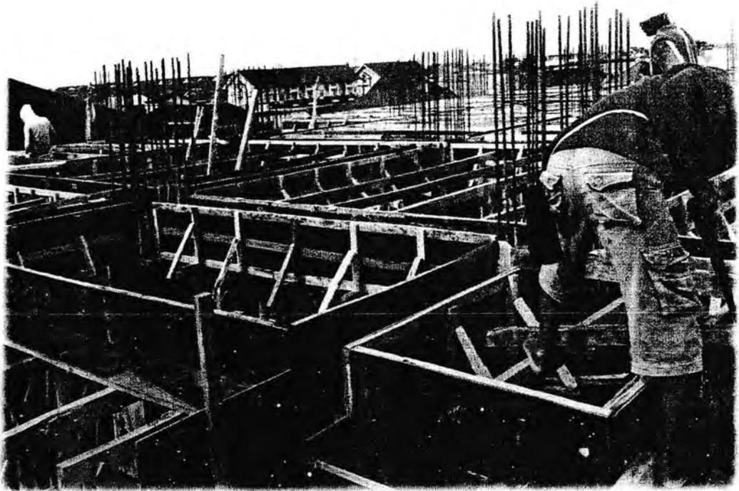
Gambar 15. Proses Bakisting Balok Tampak Atas Gedung
