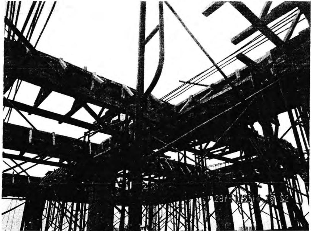
Gambar 14. Proses Bakisting Balok
