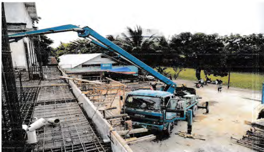
Gambar 3.2 Concrete Pump
