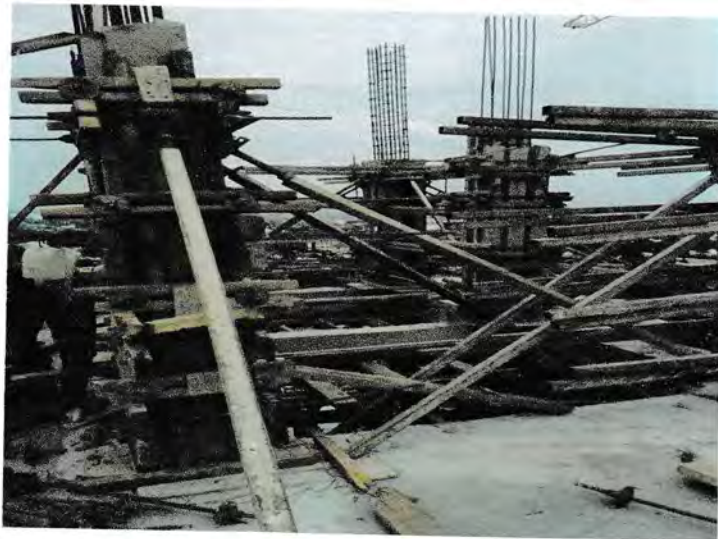
Gambar 3.2.3 : Bekisting kolom
