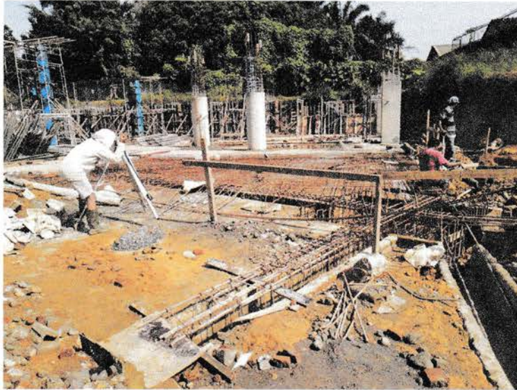
Gambar 3.2.9 Penentuan as kolom
