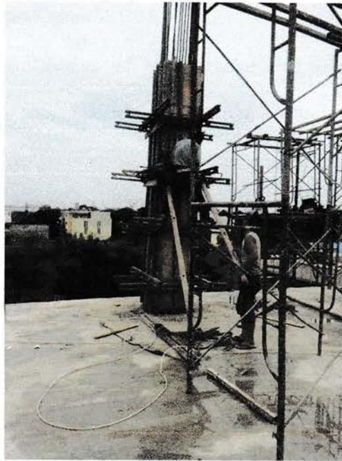
Gambar 3. Pemasangan Adjustable Kickers Bekisting
